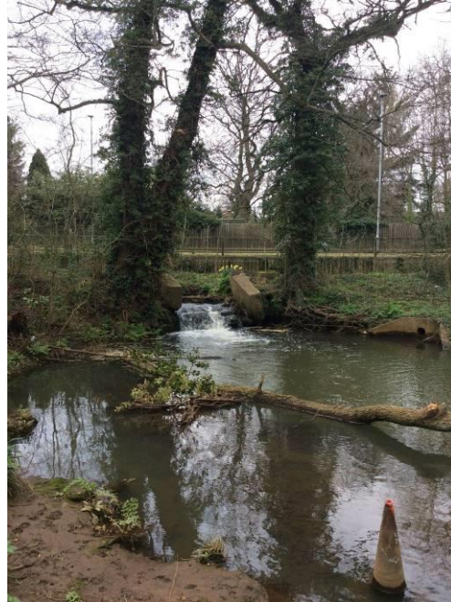
2. Weir and pool in the main channel (TN1).
