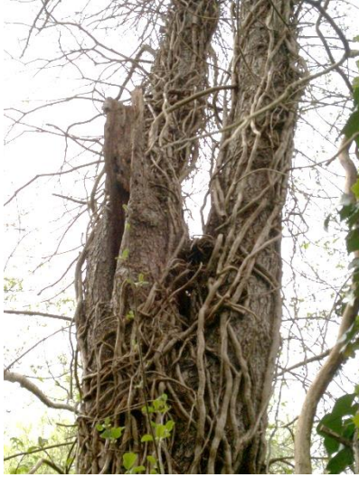
43. A tear-out and small compression fork in T27.
