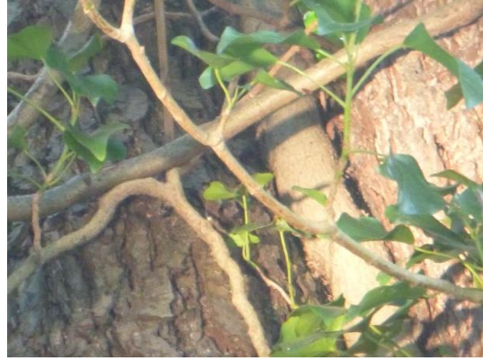
10. Potential crevice behind thick ivy stems on T5.
